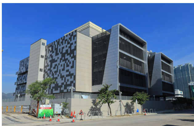
Global Switch Data Centre
