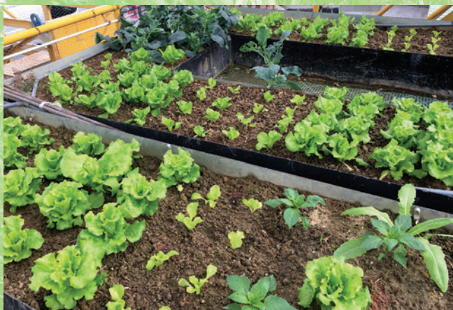
At our Hang Tau depot, vegetable beds planted on top of container offices provide both fresh food for workers and a reduction in heat transfer through the roofs
